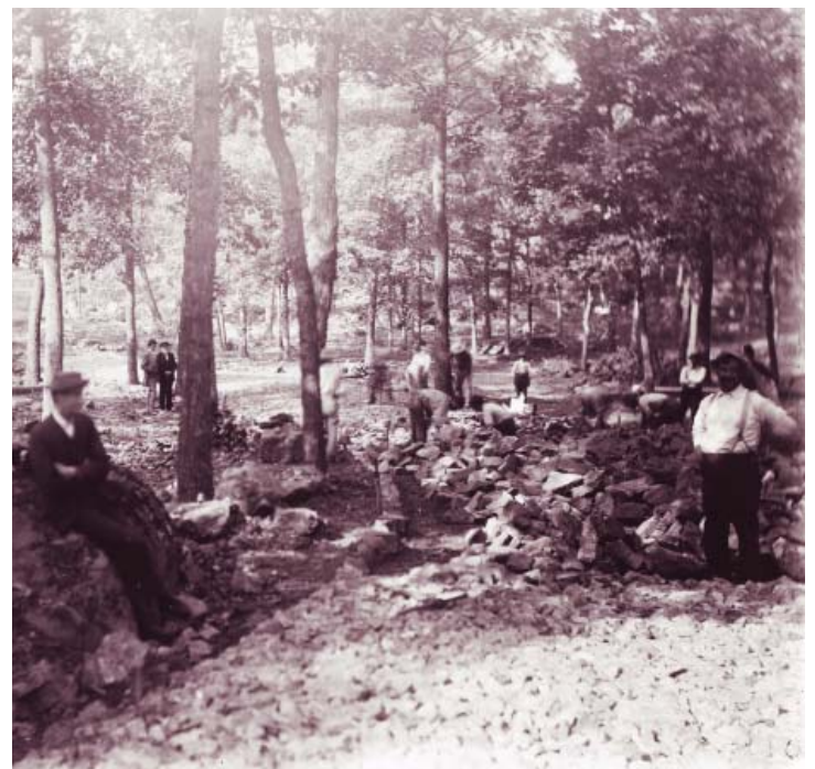
Figure 2.30. Construction of Sykes Avenue at the foot of Big Round Top, showing men laying base stones, looking in the direction of Vincent Spur. Photograph by Tipton, 1897 (GNMP Tipton Photographic Prints GETT 41136 #3098).
