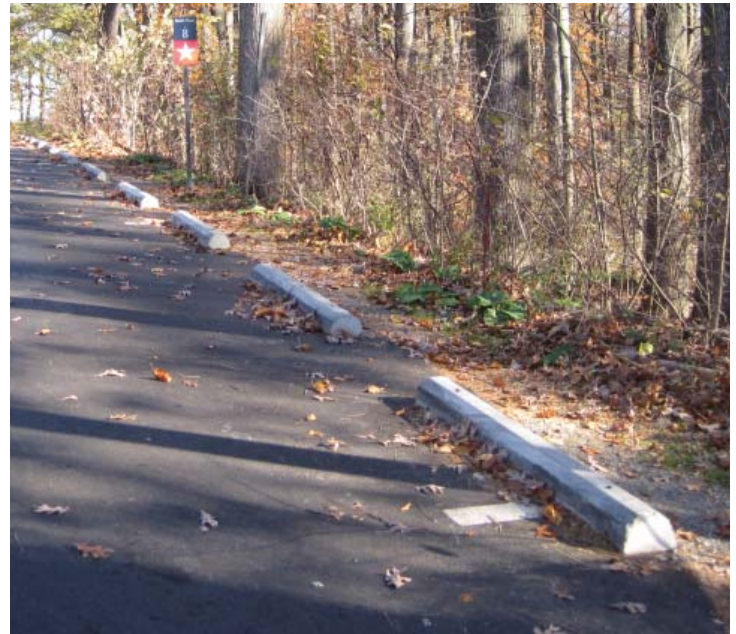
Figure 3.17. Concrete wheel stops prevent vehicles from driving off the side of Sykes Avenue and down the adjacent slope. (Photo by RHI, 2010).
