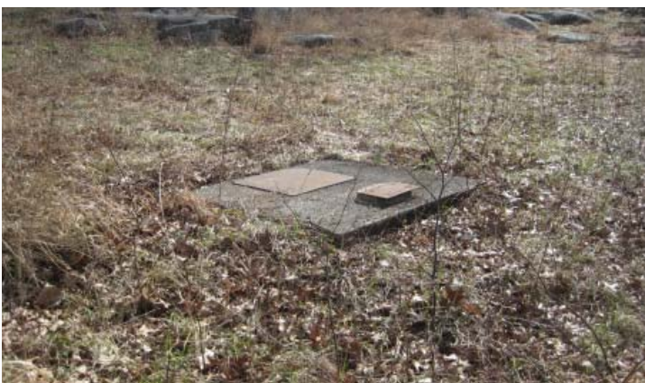
Figure 3.80. Concrete well cap near the asphalt pull-off on Warren Avenue (Photo by RHI, 2011).
