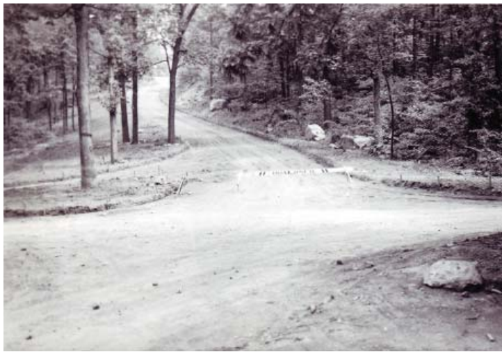
Figure 2.41. Relocating and preparing to resurface roads at the intersection of Sykes and Warren avenues, ca. 1935 (GNMP General Historic Photographic Prints GETT 41135 #SF-17M-002).
