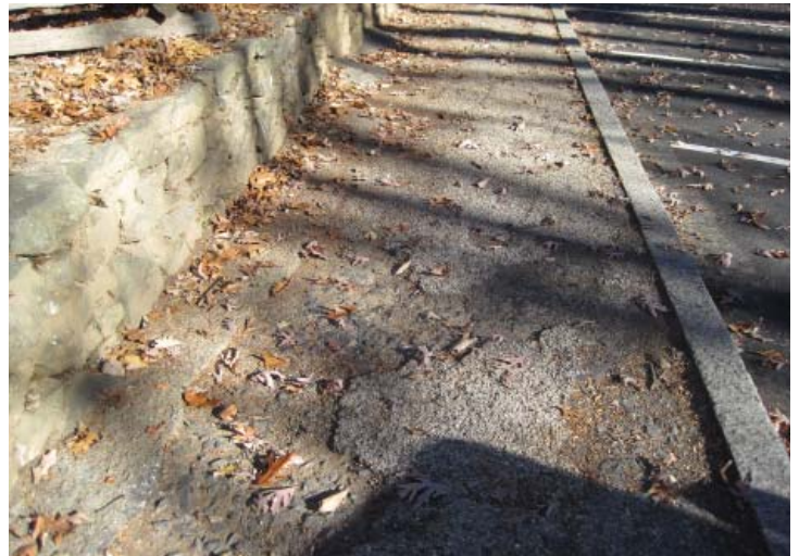
Figure 3.16. Granite curb and asphalt sidewalk at the Sykes avenue parking area (Photo by RHI, 2010).
