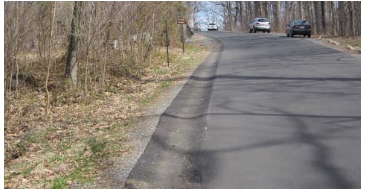
Figure 3.91. Asphalt gutter on the west side of Sykes Avenue (Photo by RHI, 2011).
