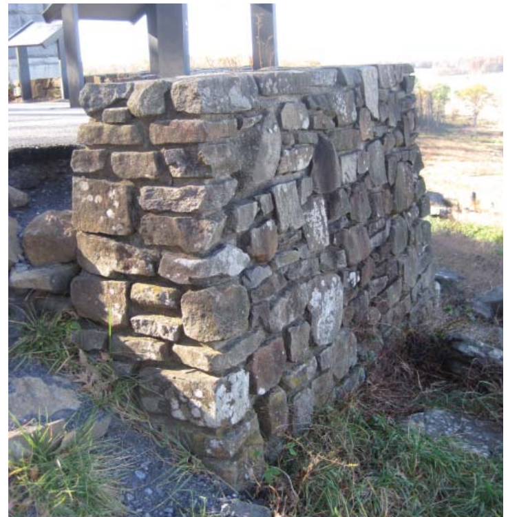
Figure 3.74. Stone and mortar retaining wall at the summit of Little Round Top (Photo by RHI, 2010).
