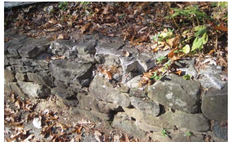
Figure 3.75. Damage to the cap of the stone and mortar retaining wall at the Sykes Avenue parking area (Photo by RHI, 2010).
