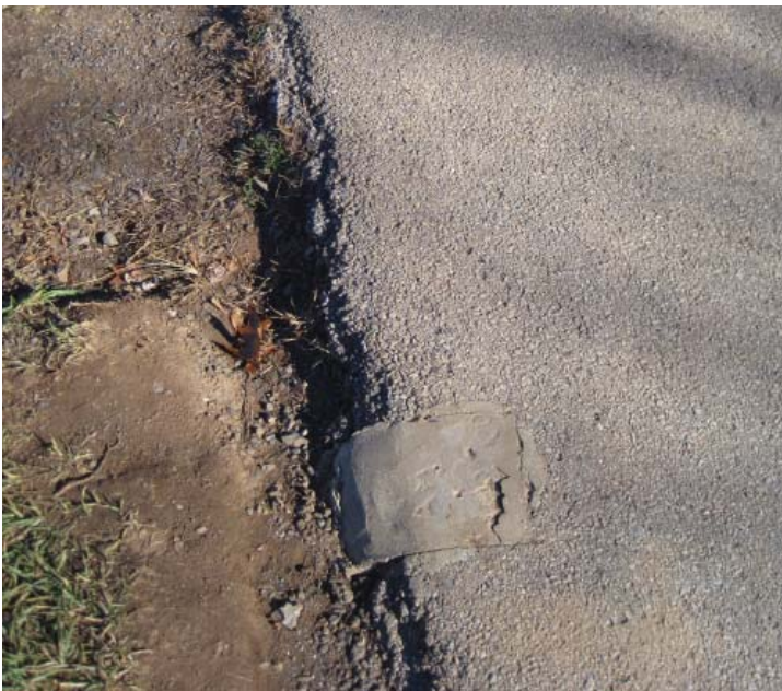
Figure 3.78. Remnant of the post-and-chain system installed to keep visitors on the asphalt paths at the summit of Little Round Top (Photo by RHI, 2010).
