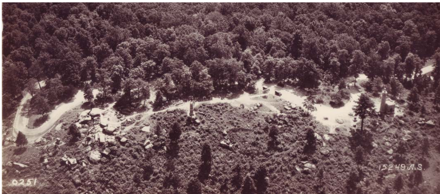
Figure 4.01. Aerial view of Little Round Top from the west, ca. 1933 (GNMP General Historic Photographic Prints GETT 41135 #SF-21P-2152).
