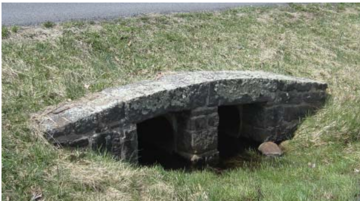
Figure 3.89. NPS Era round-topped stone culvert, constructed by the Civilian Conservation Corps (Photo by RHI, 2011).
