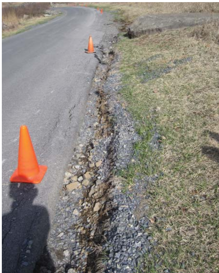
Figure 3.93. Undercutting of the roadbed along the north side of Warren Avenue has caused a partial failure of the roadway (Photo by RHI, 2011).
