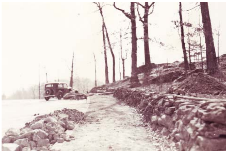
Figure 2.42. Construction of walkways and retaining wall at the Sykes Avenue parking lot on Little Round Top, ca. 1936-1937 (GNMP General Historic Photographic Prints GETT 41135 #SF-30W-093).
