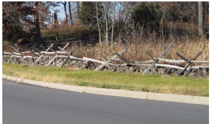
Figure 3.15. Concrete curb along the northern edge of Wheatfield Road. (Photo by RHI, 2010).
