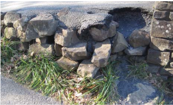
Figure 3.19. Asphalt paths show significant erosion at the edges. These paths line the summit of Little Round Top (Photo by RHI, 2010).
